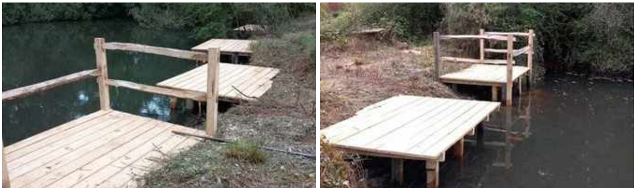
Donald's Pond with new pond dipping platforms
