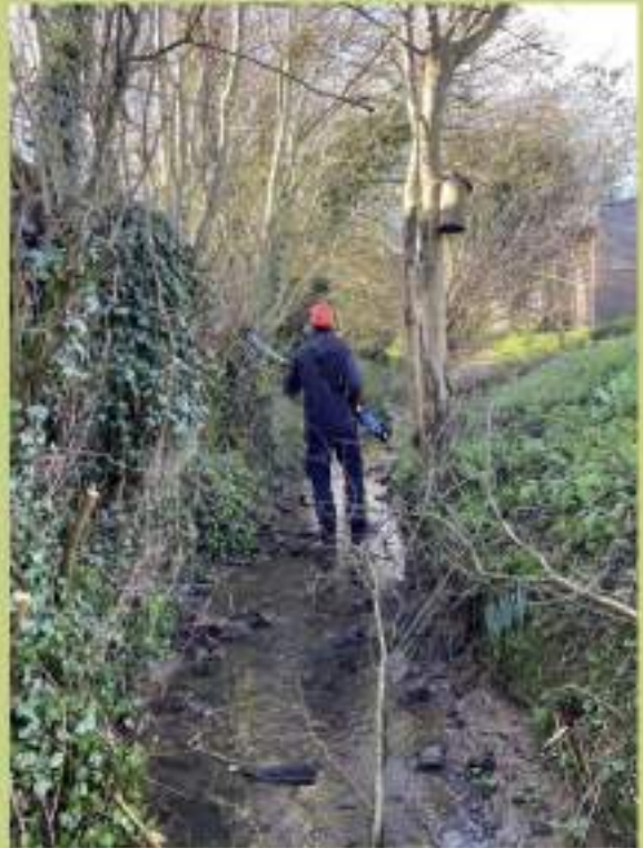
Ranger undertaking stream improvement works
