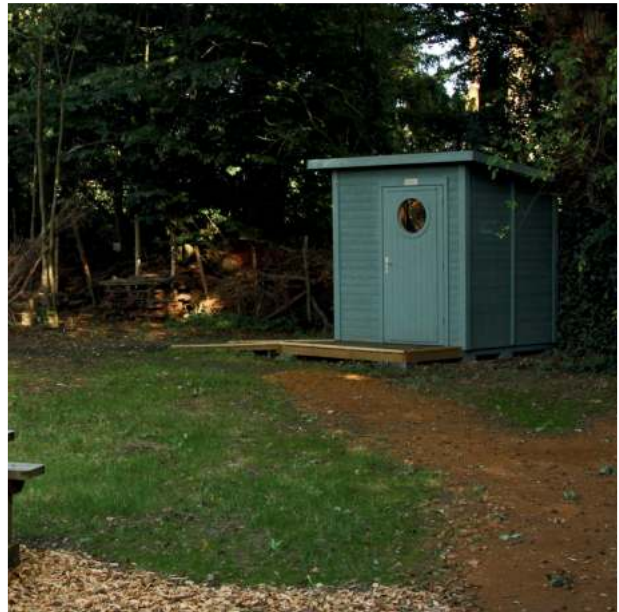
Accessible compost toilet
